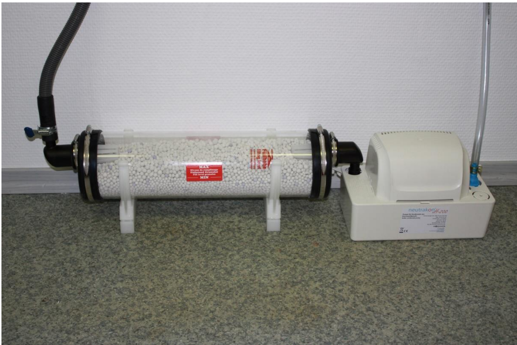
Abb. 4 / Neutralization mounted on the floor with angle nozzle and adapter for installation height discharging to a condensate pump Neutrakon pH200.
