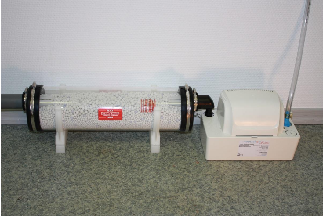
Abb. 5 / Neutralization mounted on the floor with angle nozzle and adapter for installation height discharging to a condensate pump Neutrakon pH200. Inlet DN 40
