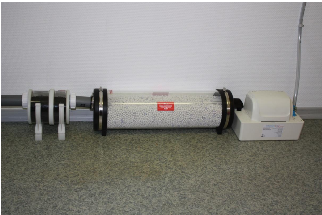
Abb. 10 / Neutralization DN 150 (N65 to N1000) with active carbon pre filter AK 1 and condensate pump Neutrakon pH200. Connection DN 40 / 90 mm pipe. AK 1 with adapter for installation height.
