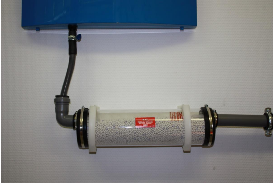
Abb. 3 / Wall mounting with HAT pipe connection (DN 40).
