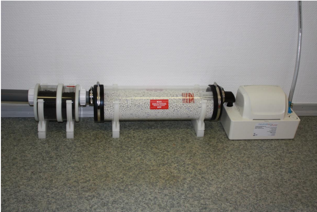
Abb. 9 / Neutralization unit Neutrakon in combination with active carbon pre filter AK1; discharge into a condensate pump with adapter for installation height
